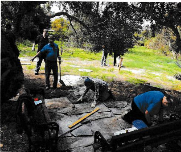
Palm and Cycad Society (SA) installing flagstone paving. EB
