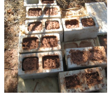
Bee wall under construction Photos by: JG, MZ & KH
