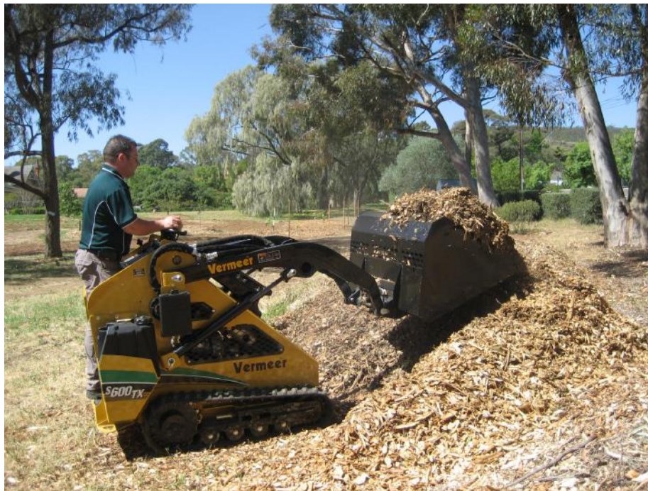
The Skid Steer in action shifting one of the many truck loads of mulch donated to the Arboretum by arboricultural industry.
